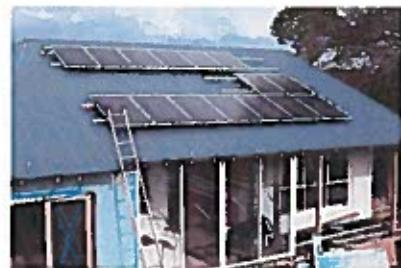
Connected at a voltage less than 60 kilovolts (kV) which may be connected in parallel operation to the utility's electric system
