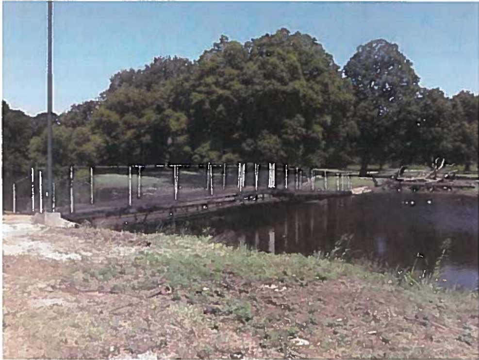
Photo No. 1: Overview of subject bridge
