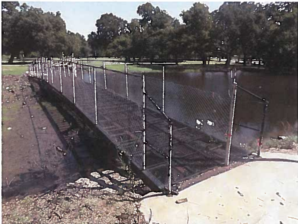
Photo No. 2: Overview of subject bridge
