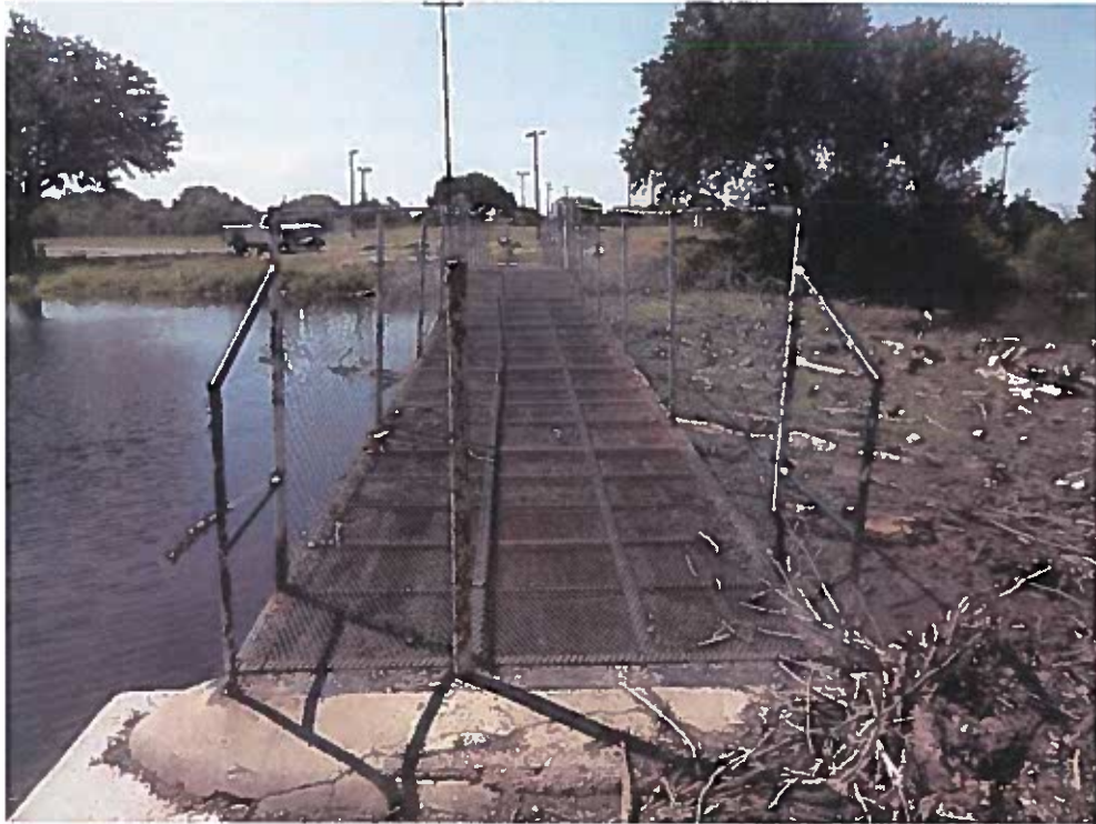
Photo No. 3: Overview of subject bridge
